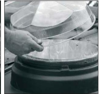
Carefully brush down the roof covering and the flashing to remove any particles of dust or dirt. Clean the dome with a soft cloth and water to ensure that the dome is free from any finger marks, dust or dirt.
