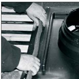
Stick the foam weathering strip to the flashing as shown below ensuring its positioned outside the weathering upstand.
