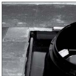
You can then cut the tiles around the ABS upstand with an angle grinder and place the tiles in position to make sure they fit.
