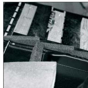
**Note:** Depending on tile type it may be necessary to trim the top foam and the foam strips either side of the flashing plate. When trimming the side strips they need to form a series of 'steps', as shown, where the tiles will sit.
