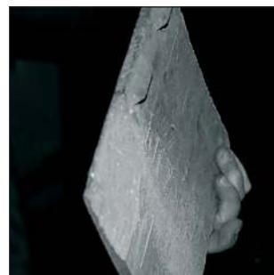
If necessary, grind off the corner nib on the back of the tiles to ensure the tiles sit correctly on top of the flashing plate.
